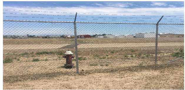
Ontario perimeter fencing
