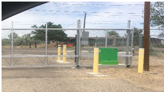
Ontario entry point access keypads
