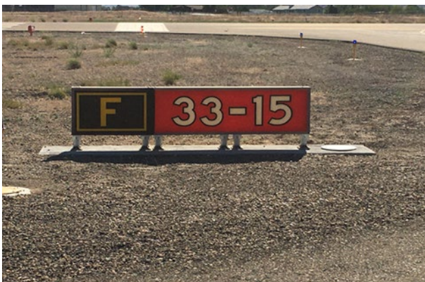
Foxtrot Taxiway / Runway 33/15 location sign
